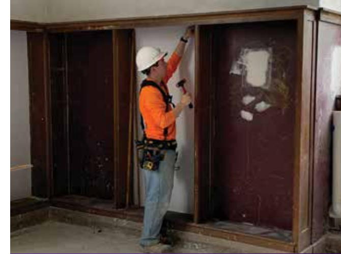
The original bookshelves located in the east and west alcoves of the Great Room are in the process of being restored. After the bookshelves are repaired, they are stripped and then varnished by hand.
